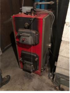
View of furnace in basement. Gaskets inside assumed asbestos (friable)
