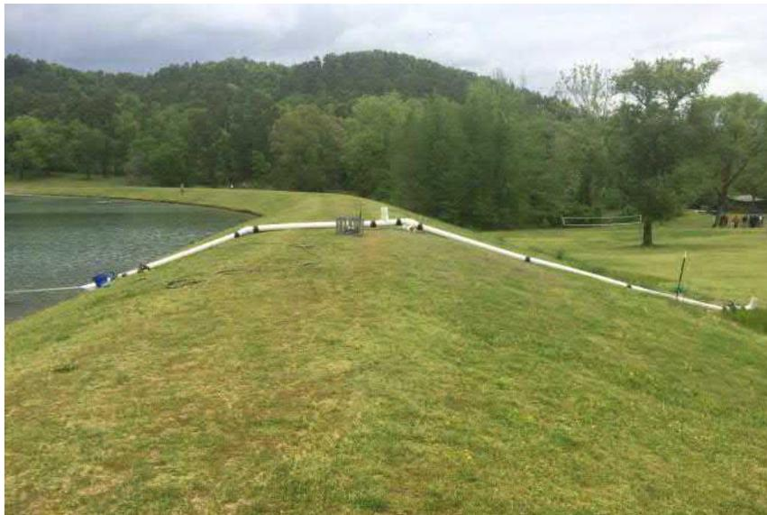
FIGURE 11 - PHOTO OF SIPHON DRAIN ON DAM
