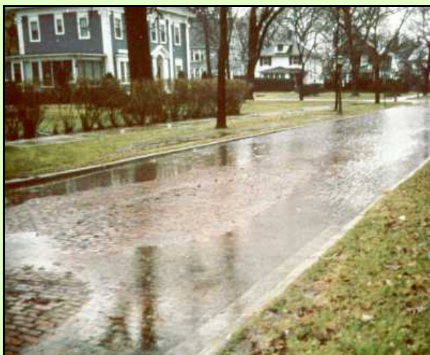
Figure 1. Runoff temporarily stored on a street surface.
